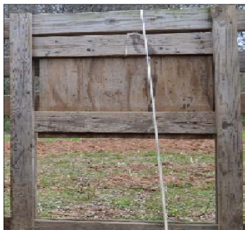
Figure 26: An example of a common wooden guillotine gate. Photo taken by M.T. Mengak.
