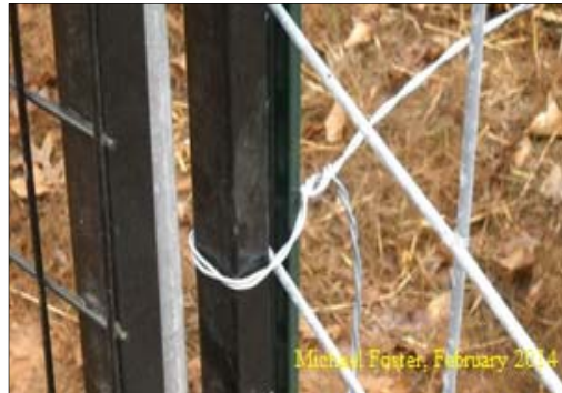
Figure 48: Steel T-Post wired to a typical guillotine door.
